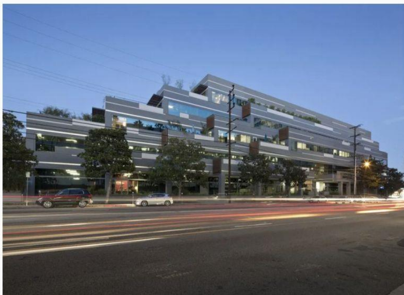
LA office building at 1640 Sepulveda Blvd. (Harbor Associates)
